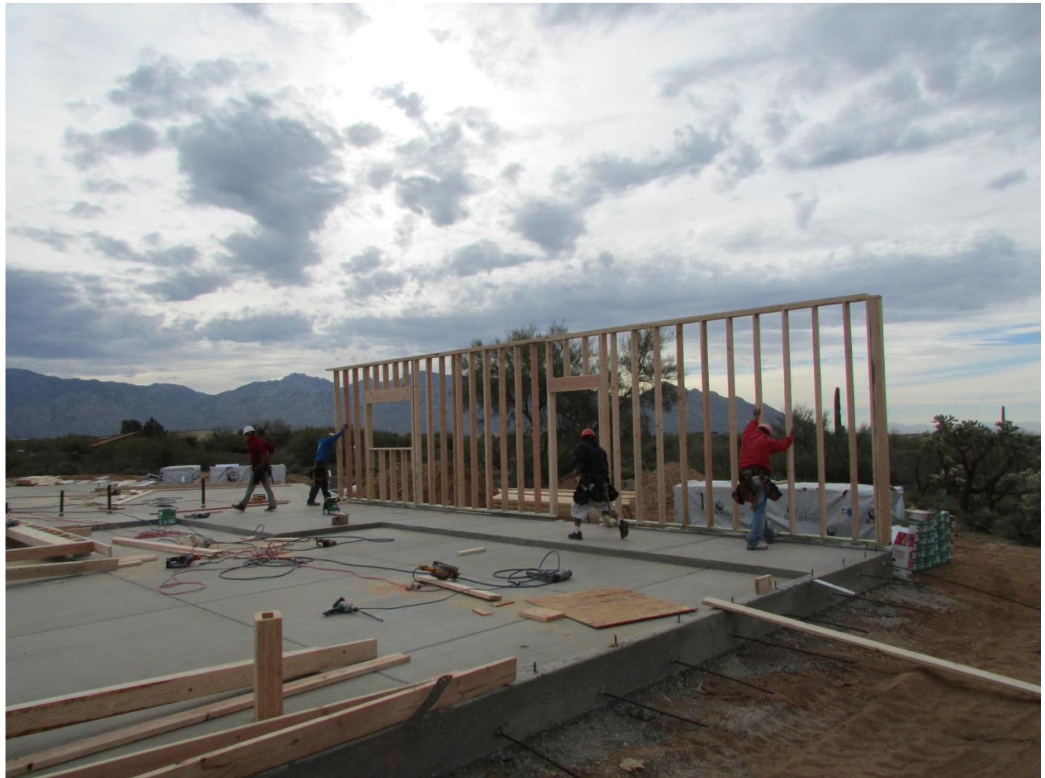
First Wall Up!
