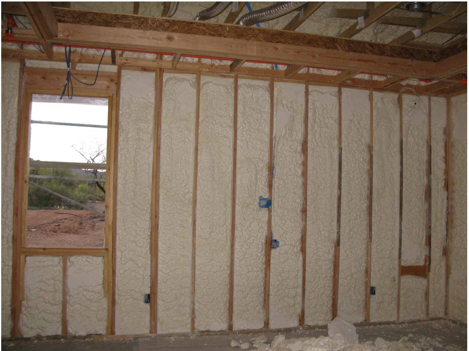
Open-cell foam was used for insulation.
