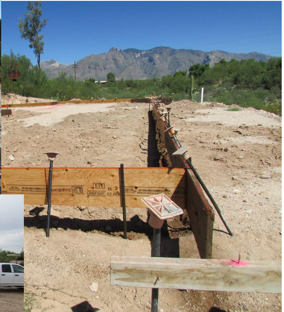
Laying out the foundation
