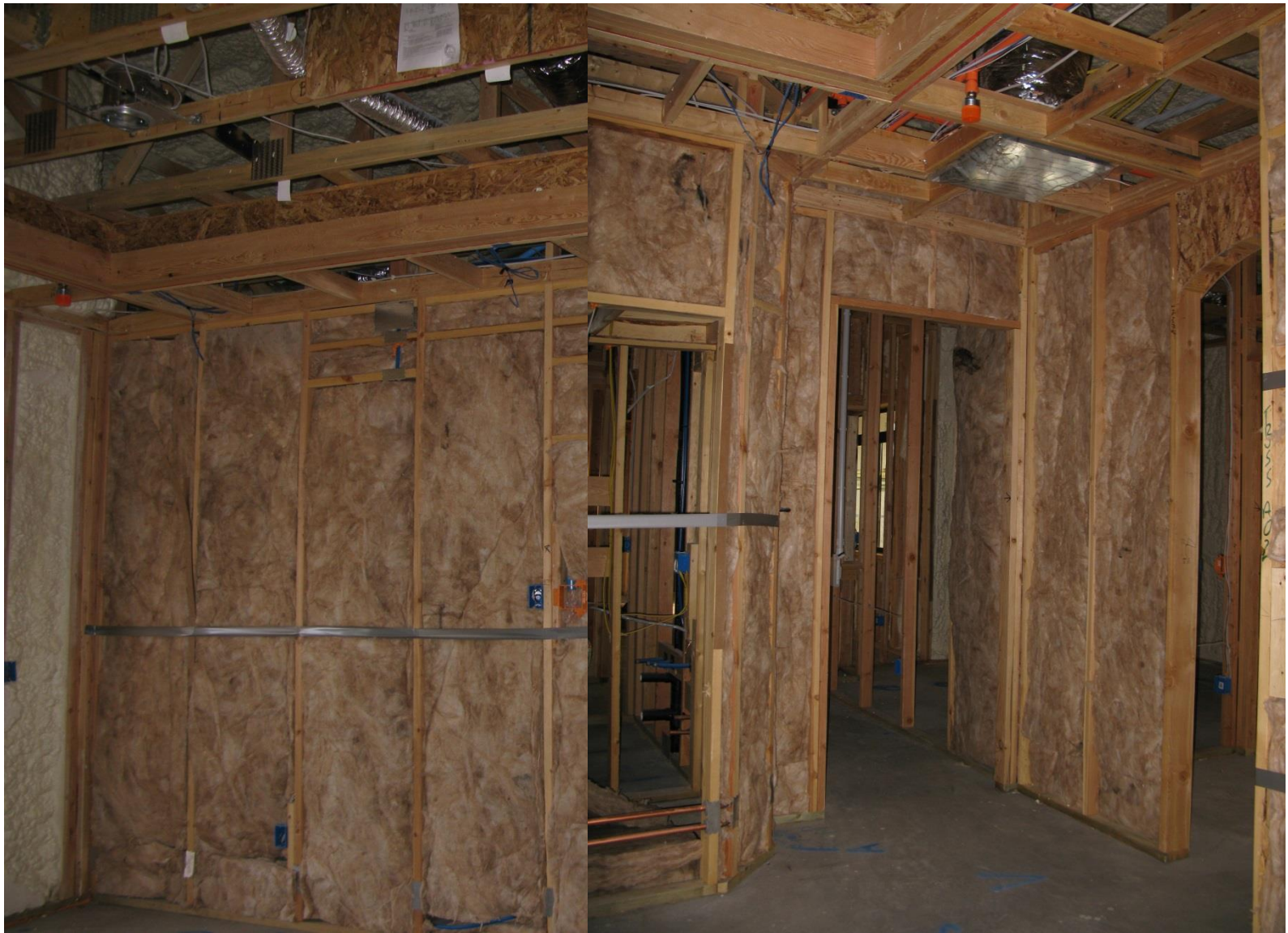
Roxul was used as a sound barrier in several interior walls.
